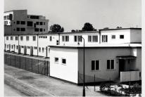
Designers: Ludwig Moshamer (no. 10-12), Heinrich Lauterbach (no. 13-15). Moritz Hadda (no. 16–17), Paul Häusler (no. 18–20), Theo Effenberger (no. 21-22) **Construction:** reinforced concrete framework filled with cellular concrete hollow bricks (12×14×25 cm) (no. 10-12), wall constructed of slag bricks (load bearing walls between the sections, 25 cm thick) (no. 13-15), reinforced
